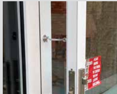
Latch added to door to avoid closing unexpectedly
